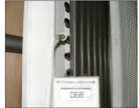
Figure 1: Commissioning a chilled beam by means of measuring the static pressure
